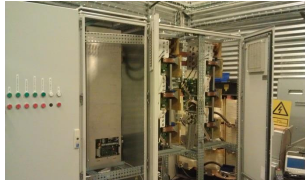
(b) A 1-MW power stack test platform.
