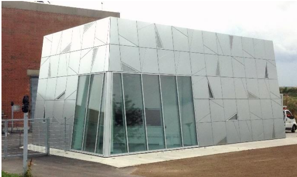
(a) The Medium Voltage Laboratory for testing of next-generation medium-voltage power converters up to 20 kV/2 MVA in a safe and controlled environment.
